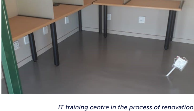
IT training centre in the process of renovation.
